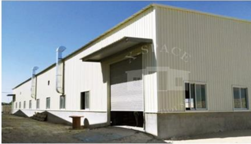
Qatar warehouse house
